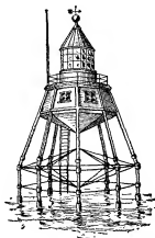
FIG. 19.—Maplin Pile Lighthouse.
